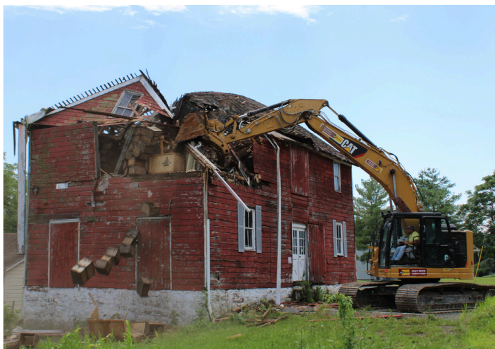
Photo of Cider Mill demolition on July 17 th , 2026
