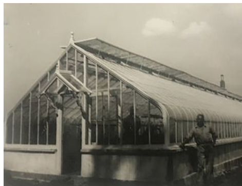
Photo of the first glass-greenhouse that we're trying to save
